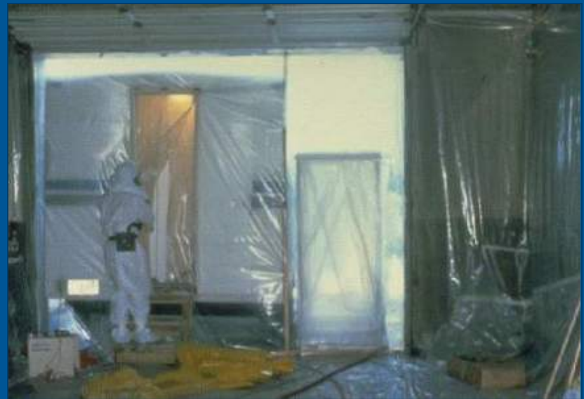
Asbestos abatement area contained and enclosed
