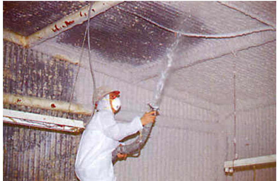
Structural Steel and Deck Coating
