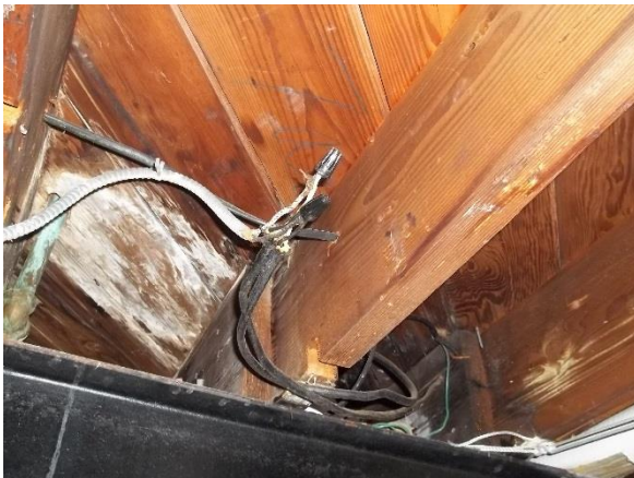
Old Administration Building (101T) – Sample of Old Basement Office Wiring on West End [Area of possible asbestos containing material. WAT 07-29-2016 sample indicated non-asbestos material.]
