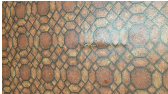
Culture Building (102T) – Floor Covering Crack Detail in Classroom 1
