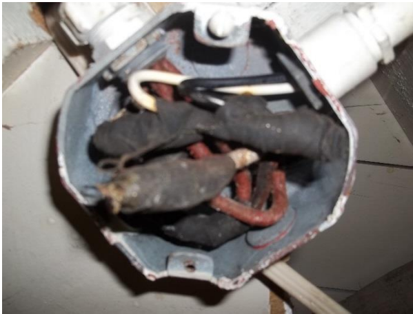
Old Administration Building (101T) – Sample of Old Basement Office Wiring on West End [Area of possible asbestos containing material]
