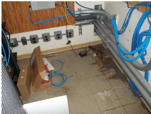
Old Administration Building (101T) – SE Corner Basement Office 6 [9" floor tiles and mastic of 3% Chrysotile]
